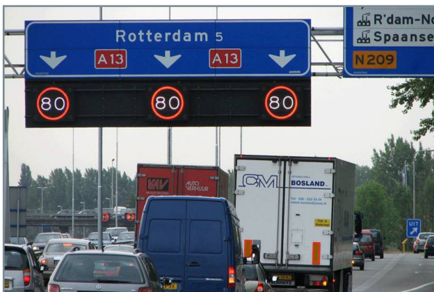
Limited variable message sign, lane control signs
