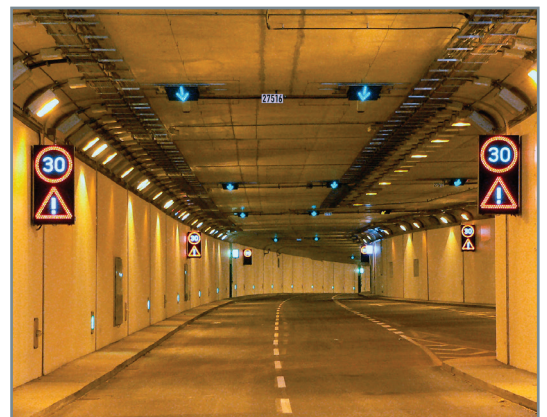
Variable message sign in tunnel, limited sign combination, "LIFE" lane control sign for mounting on tunnel ceiling (reduced total height) Germany
